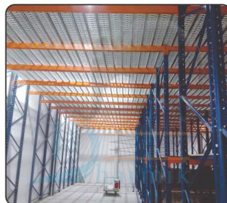
Cold Storage Rack
