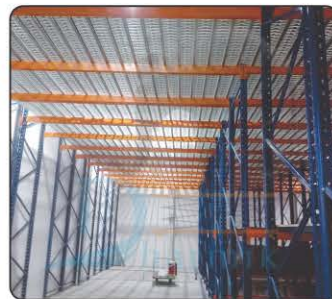
Cold Storage Rack
